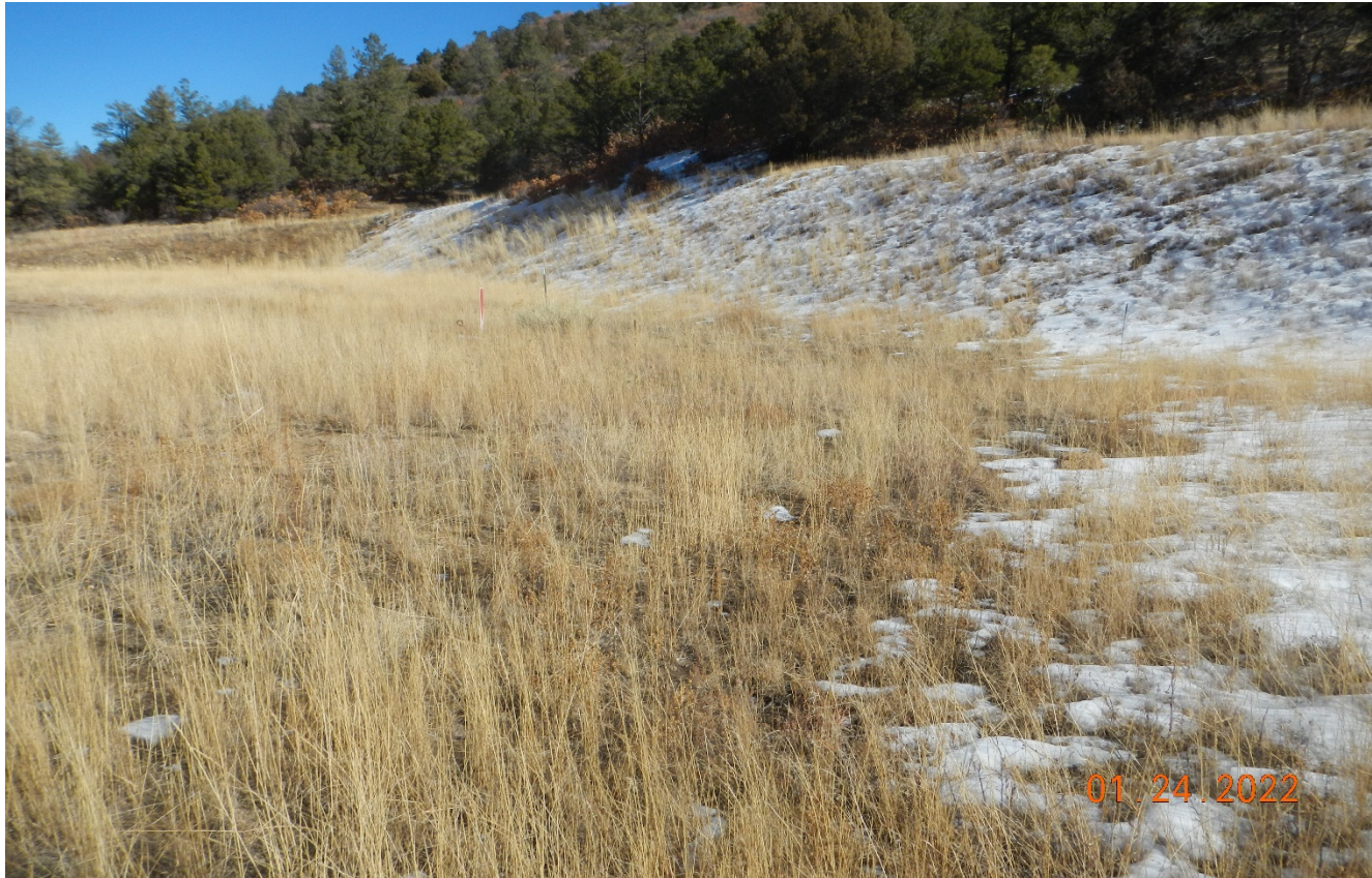
Photo 2. Facing east toward the cut slope. The vegetation is well established throughout the location.
