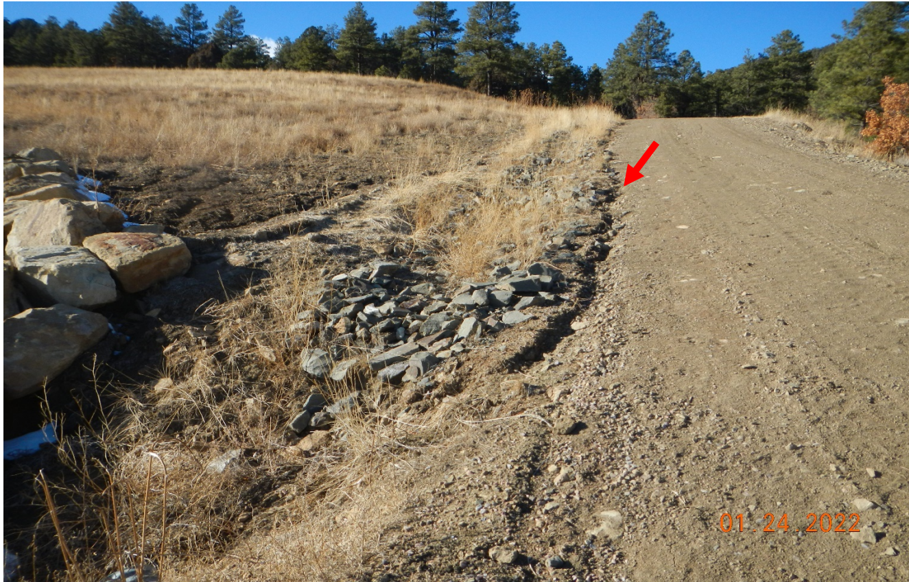
Photo 3. There is rock rip/rap placed along the roadside. It appears stormwater erosion is occurring along the side of the rip/rap which will need maintenance.
