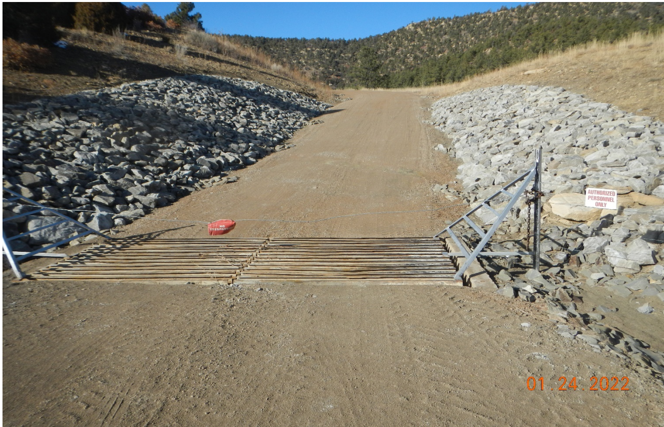
Photo 1. Facing north at the beginning of the access road. The cattleguard has been cleaned out and maintained. There is rock rip/rap installed along the road side and additional roadbase has been spread along the road.
