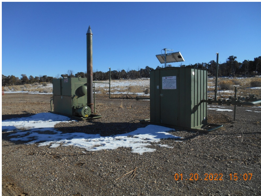
Separator and meter housing
