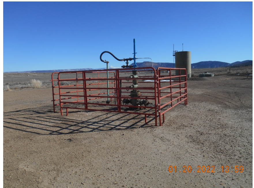
Wellhead with fence
