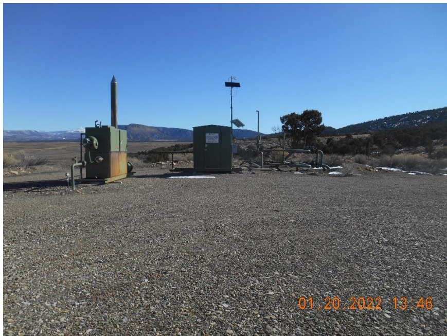
Separator and Meter housing
