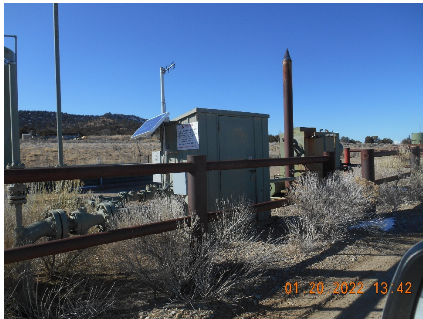
Separator and Meter Housing
