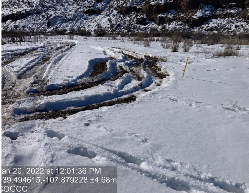
Lack of stabilization/compaction
