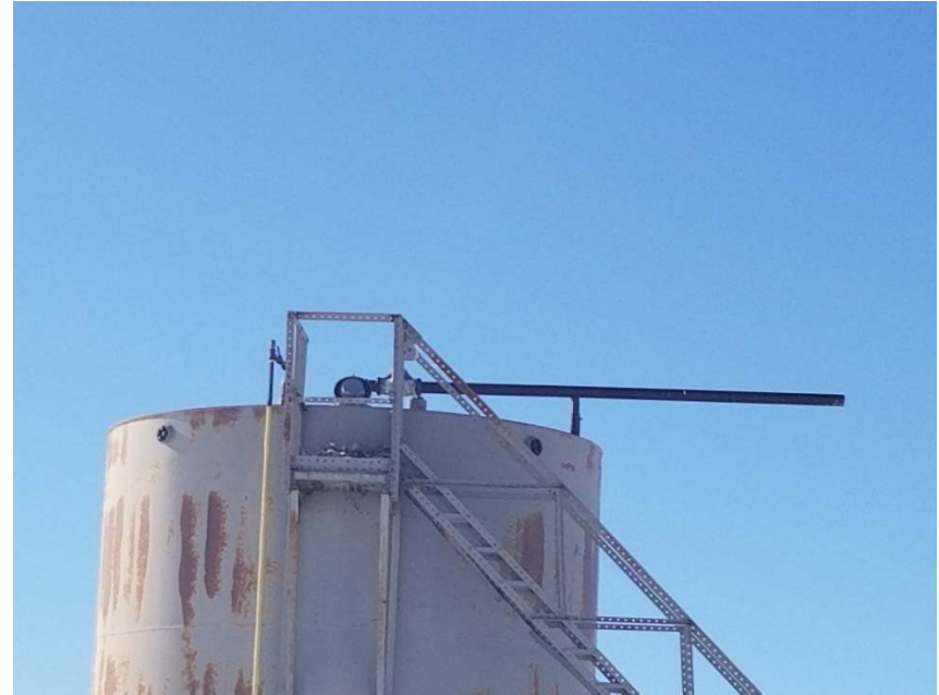
Photo 4. Close up of Photo 3, open gauge hatch on crude oil tank.
