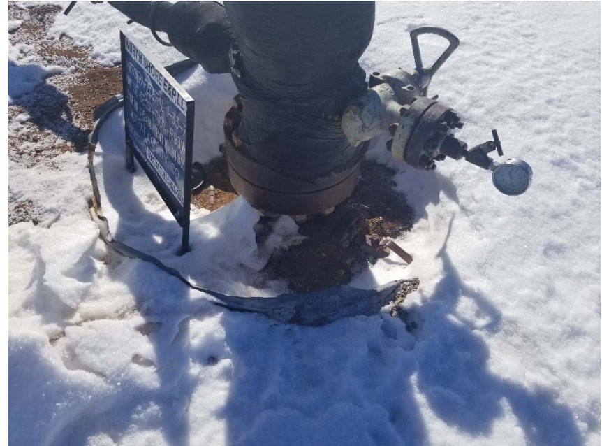
Photo 2. No bradenhead access apparent.
