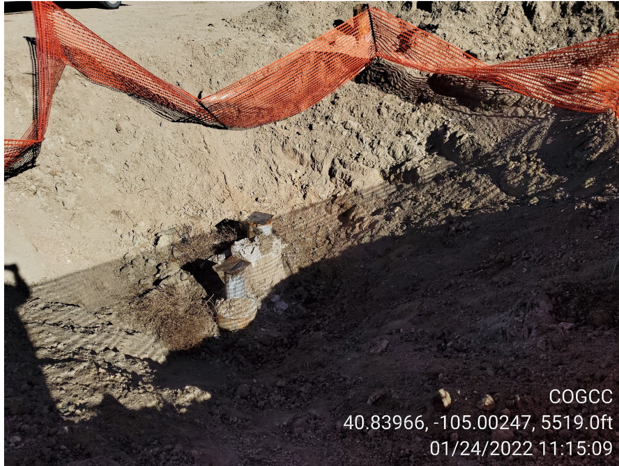
Photo 2 Well Excavation, cut & capped well
