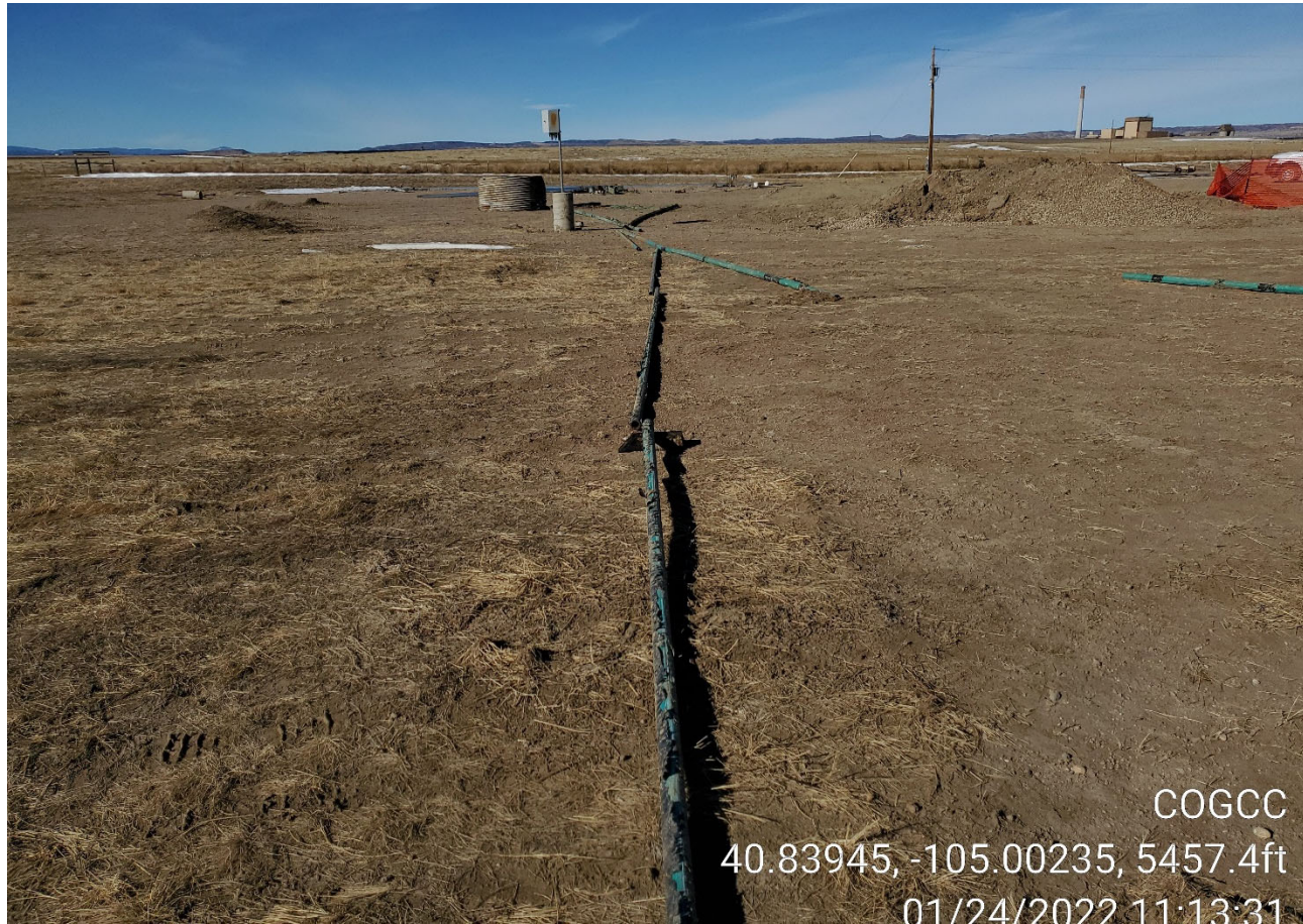
Photo 1 Removed well flowline
