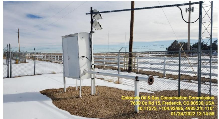
Photo 5 Produced Water vault, flow line valves
