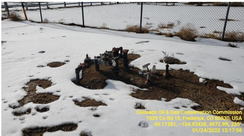
Photo 11 Flow line manifold.
