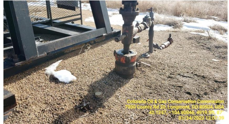
Photo 5 Bradenhead does not appear to be plumbed to surface
