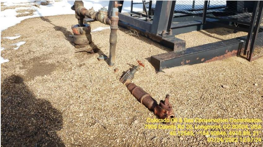
**Photo 7 Bradenhead does not appear to be plumbed to surface**
