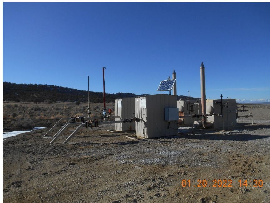
Separators and Meter housings
