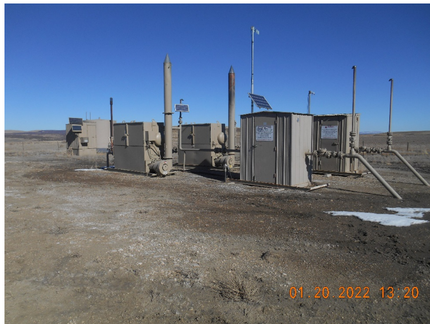
Separators and Meter housings
