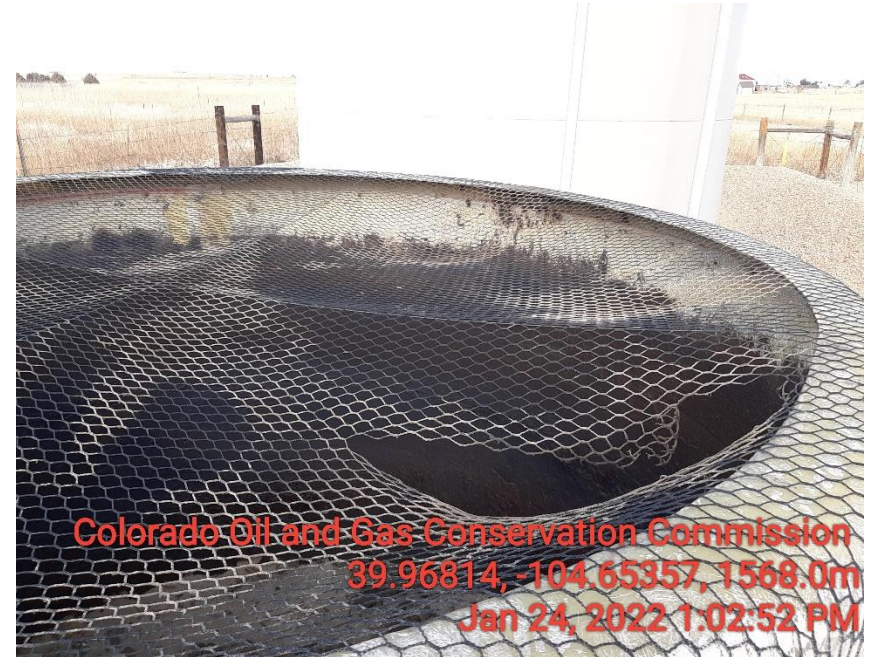
Photo 4 Bird netting on produced water tank in disrepair.
