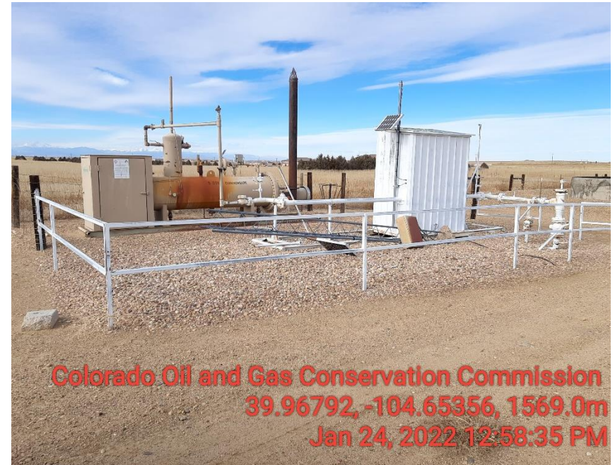
Photo 2 Production equipment. Unused equipment communication tower laying on ground
