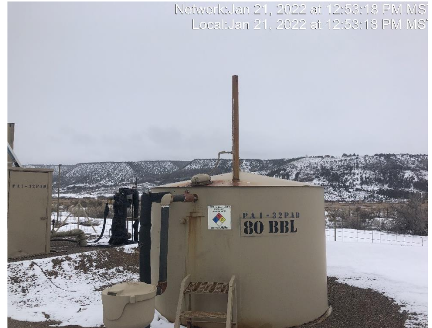
Photo #5759 Vent pipe on tank open ended.
