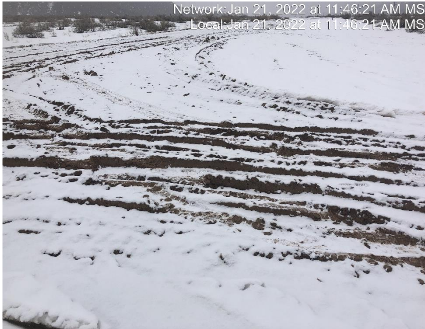
Photo #5753 Insufficient tracking BMP at entrance to location.
