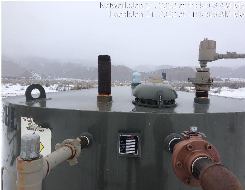
Photo #5750 Vent pipe on tank open ended.
