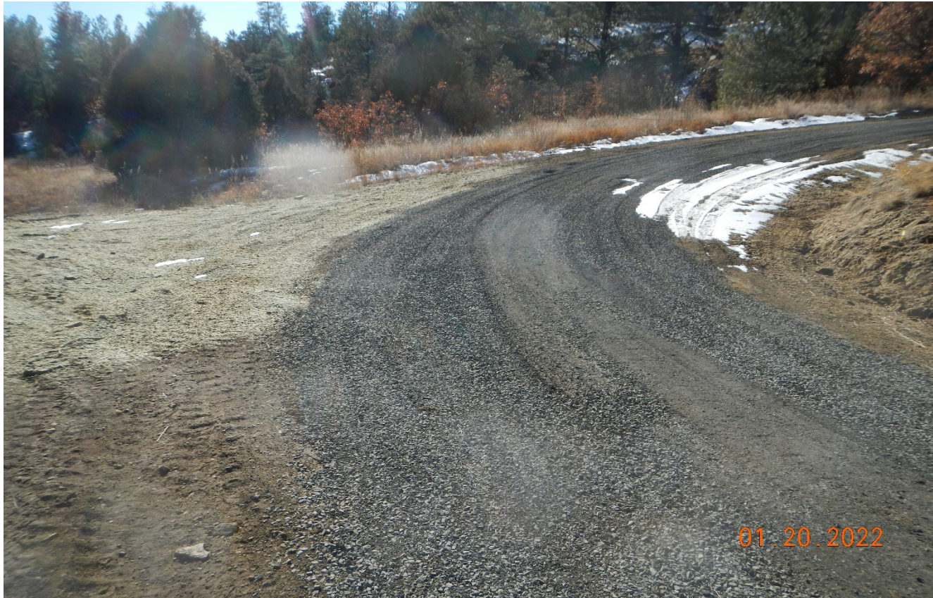
Photo 2. Facing southwest toward the access road near the location. The disturbance area has been reclaimed and gravel was spread along this area of the road.
