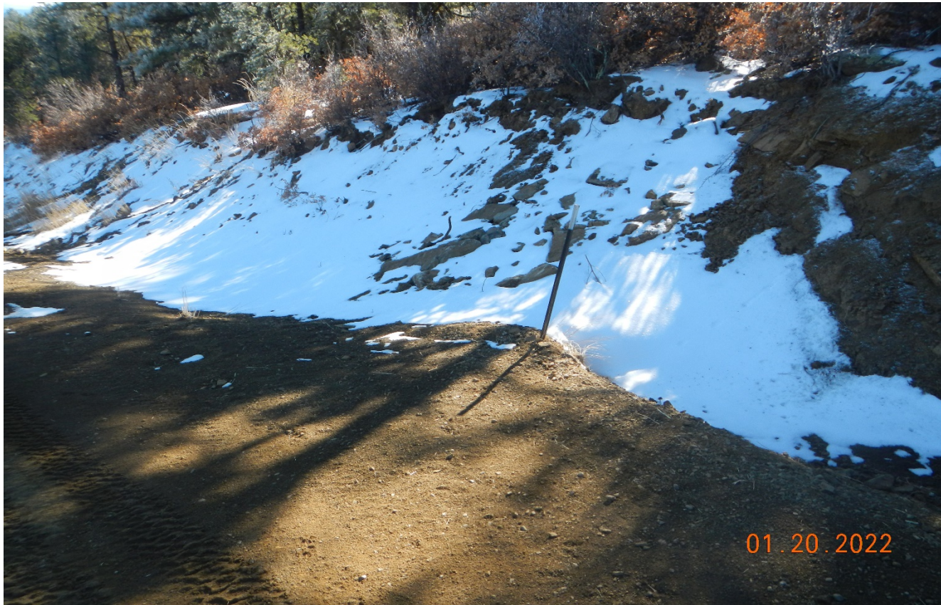
Photo 2. The erosion gully has been repaired and armored with rock rip/rap.
