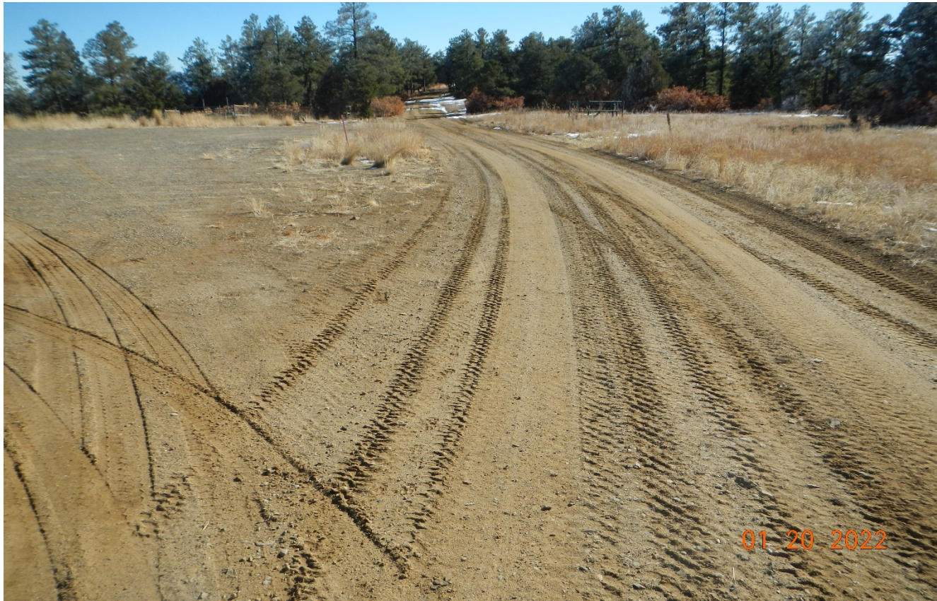
Photo 2. Facing southeast along the access road.
