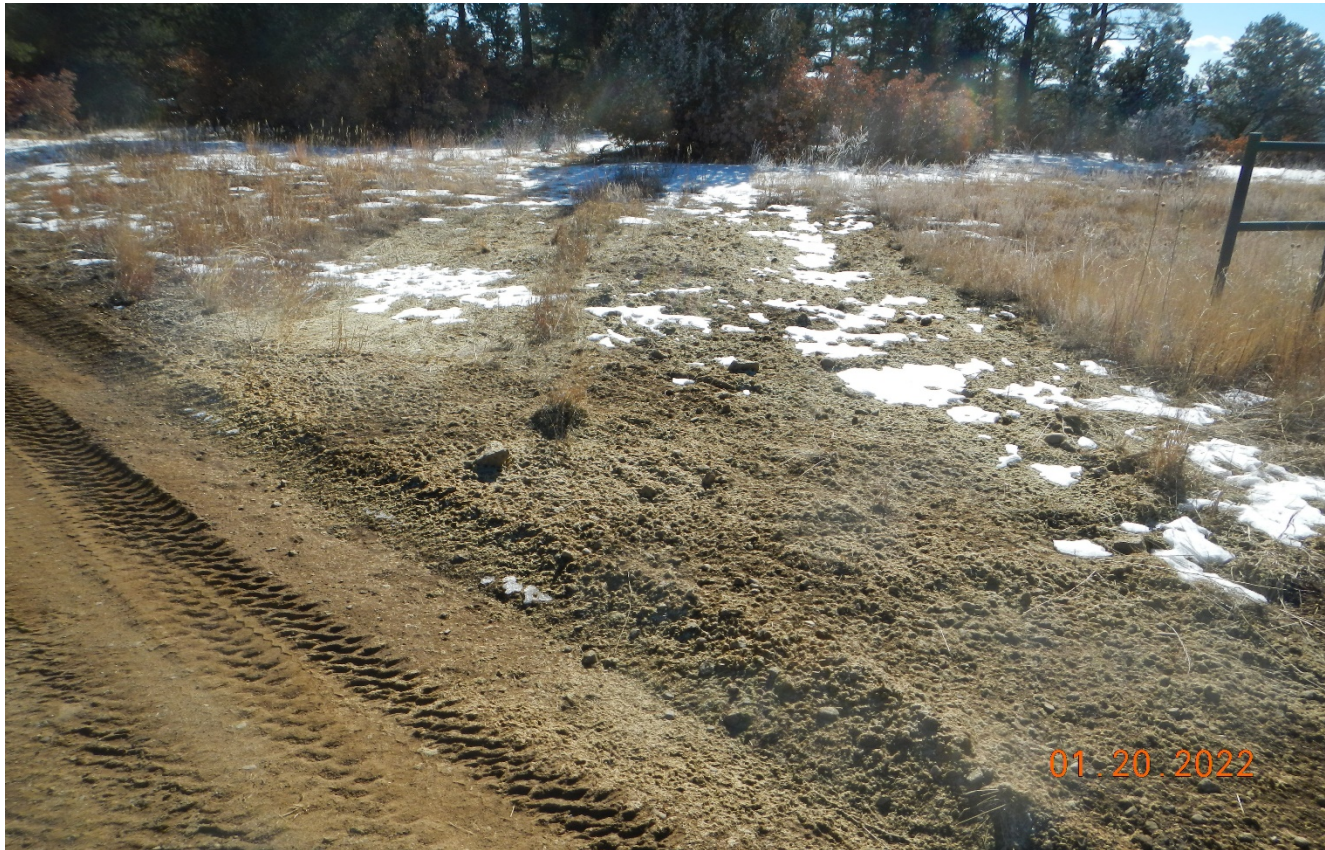
Photo 3. The ditch disturbance has been repaired and reclaimed.
