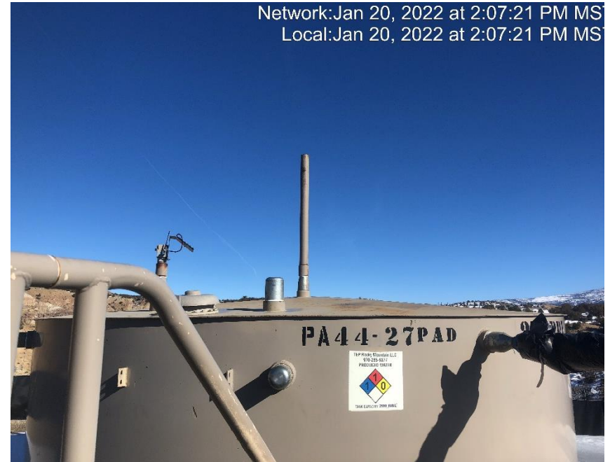
Photo #5745 Vent pipe on tank open ended.
