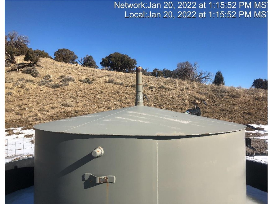
Photo #5738 Vent pipe on tank open ended.
