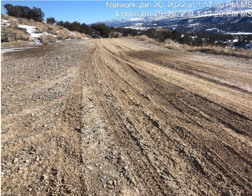
Photo #5742 Insufficient tracking BMP at entrance to location.
