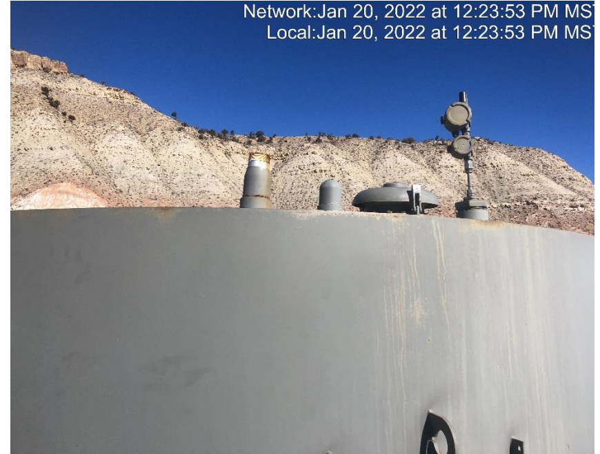
Photo #5732 Vent pipe on tank open ended.
