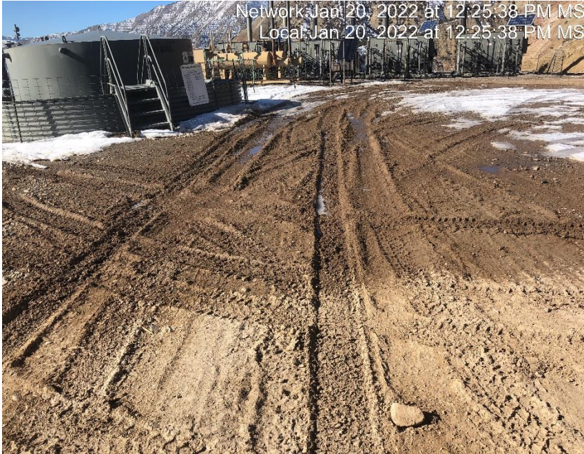
Photo #5734 Location lacks stabilization.
