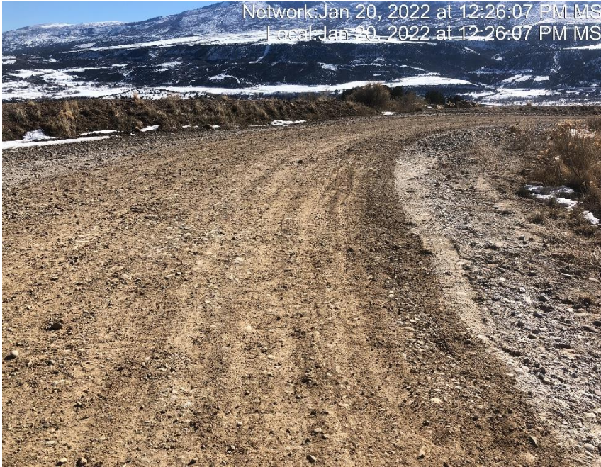
Photo #5736 Insufficient tracking BMP at entrance to location.
