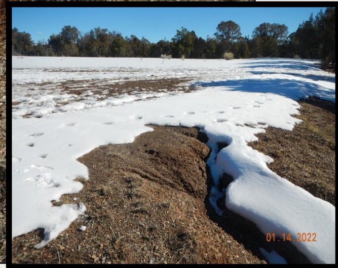
Photo 3. View of erosional channeling approximately 2ft wide and deep observed within the southern project area. Inset shows area where concentrated stormwater flows off of the southern fill slope.
