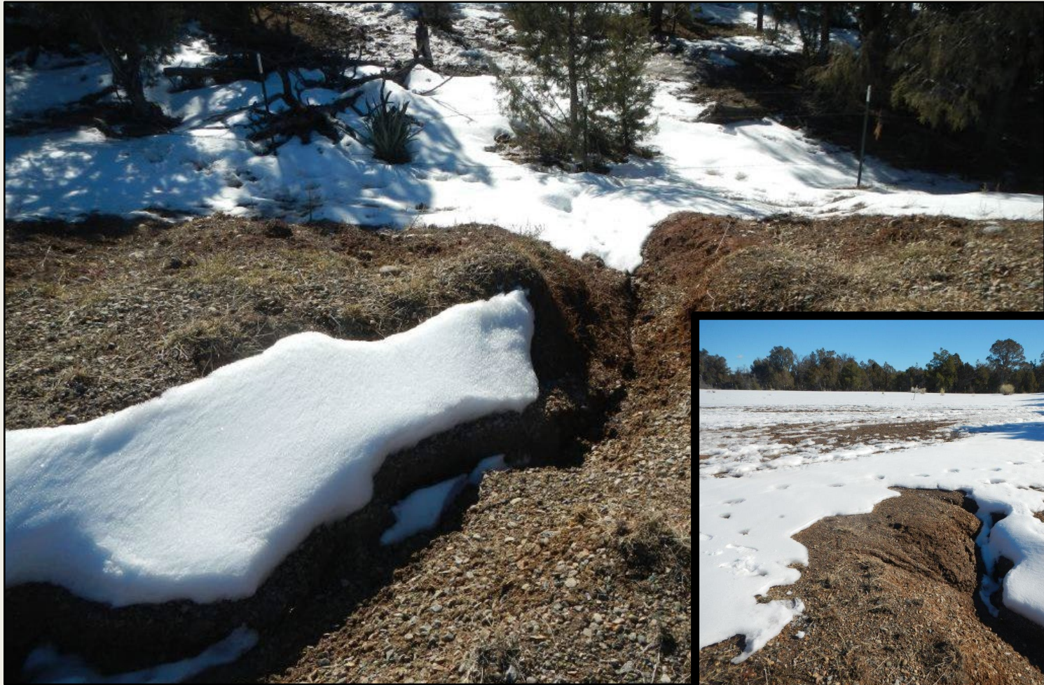
Photo 3. View of erosional channeling approximately 2ft wide and deep observed within the southern project area. Inset shows area where concentrated stormwater flows off of the southern fill slope.
