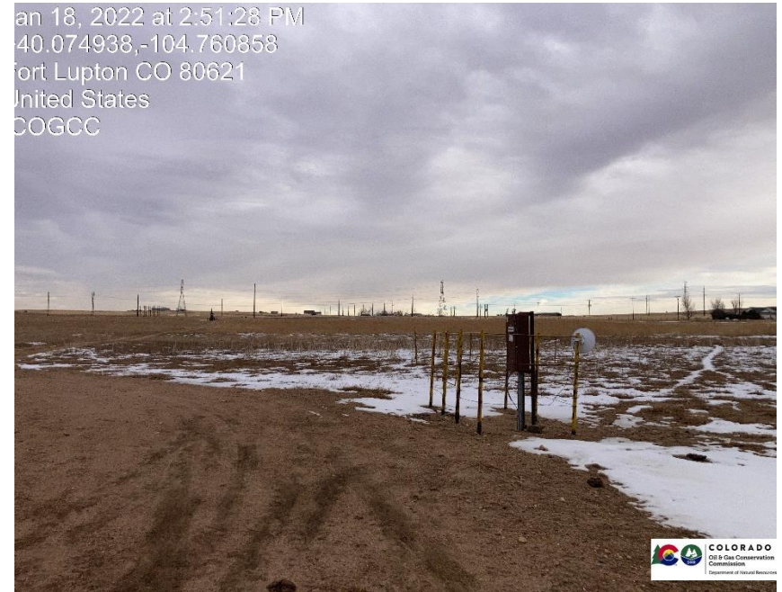
Pic 2 electric equipment.
