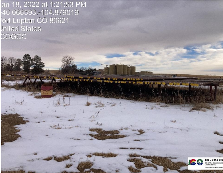
Pic 3 tubing being stored on location
