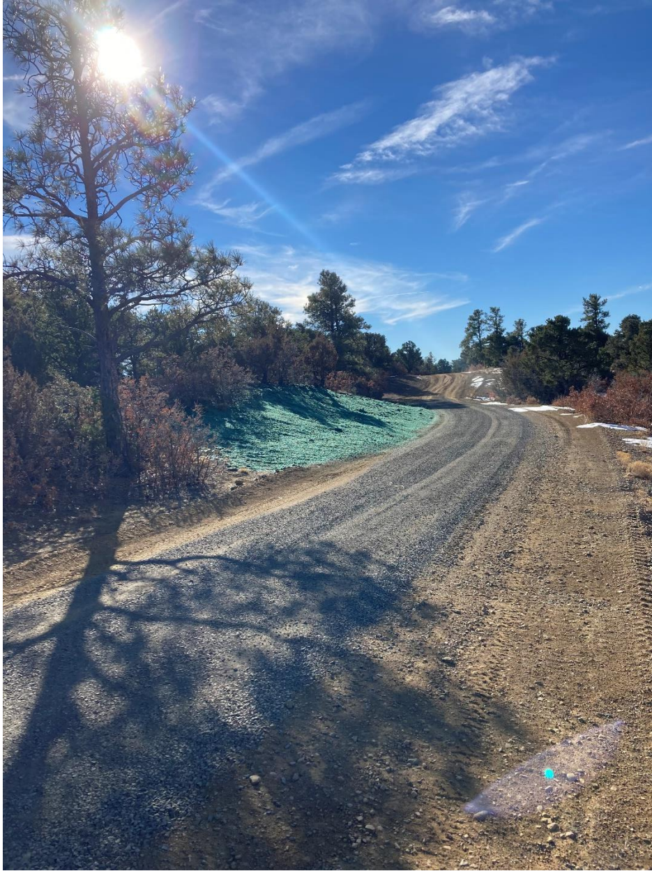
Reseed and stabilized to prevent erosion to comply with Rule 1003
