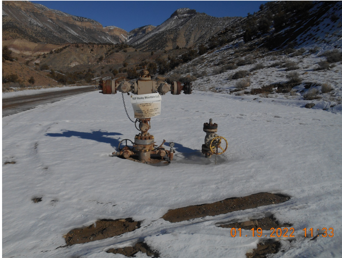
Injection wellhead. Temporarily abandoned.
