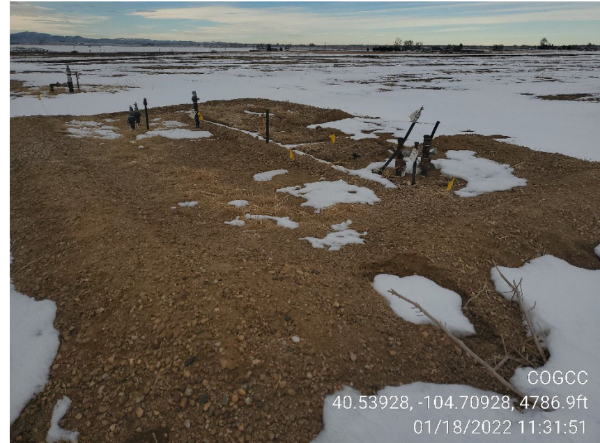
Photo 4 Separator removed on west side of tank battery and unused flowline risers
