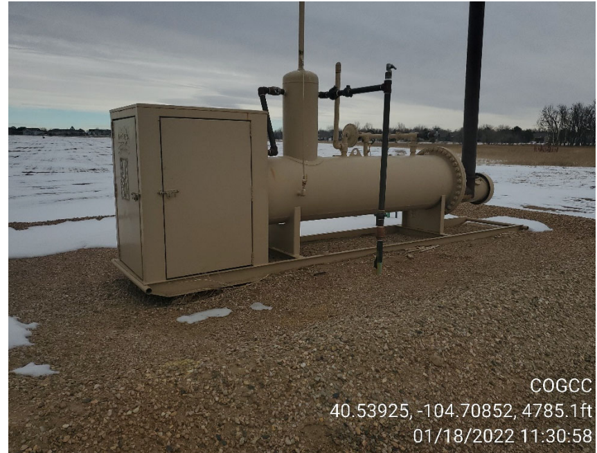
Photo 2 Separator on east end of location
