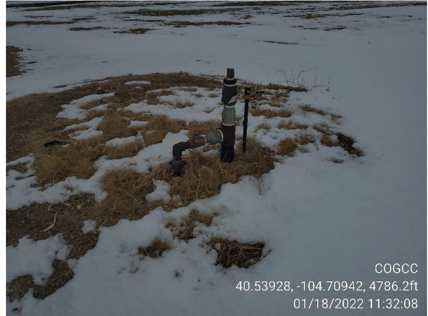
Photo 6 Unused flowline riser on west side of tank battery
