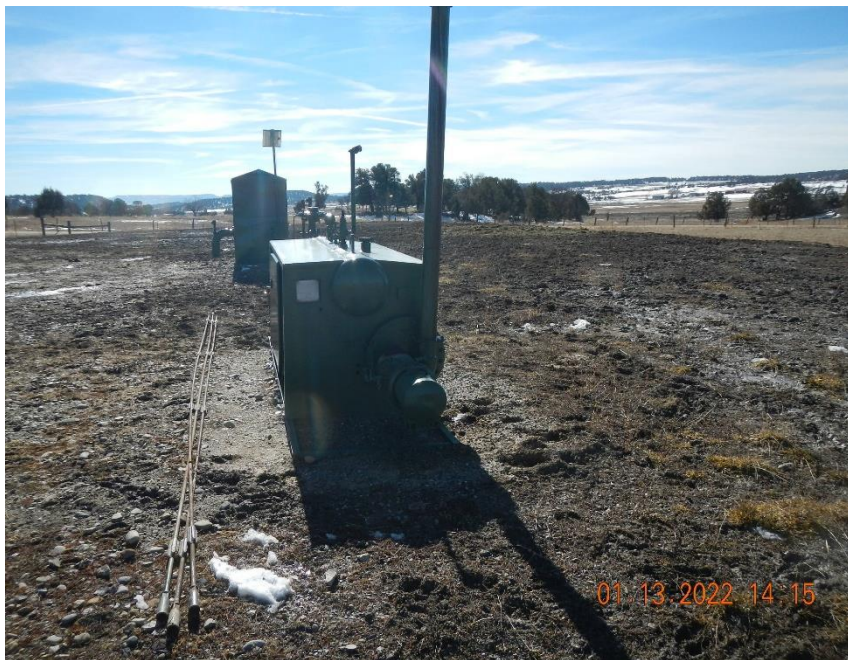
Unused equipment near separator.
