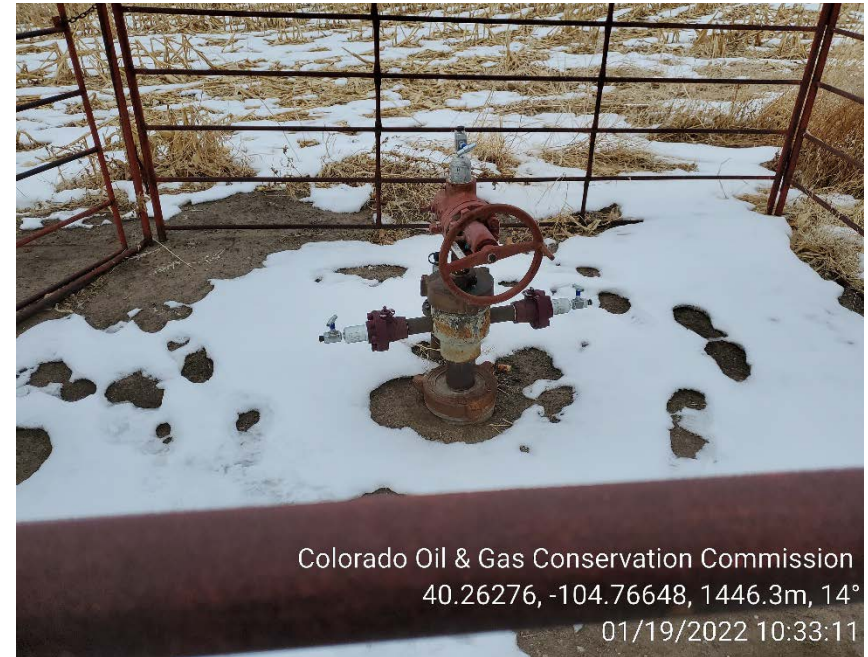
Temporarily abandoned wellhead
