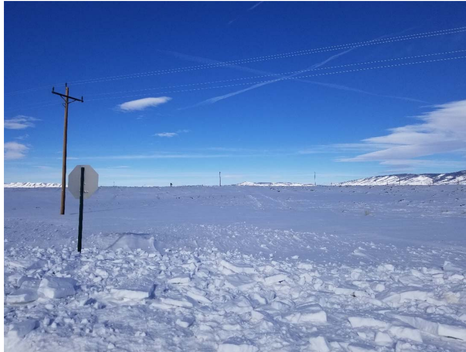
Photo 1. Access road not maintained for winter. Inspector unable to access location.
