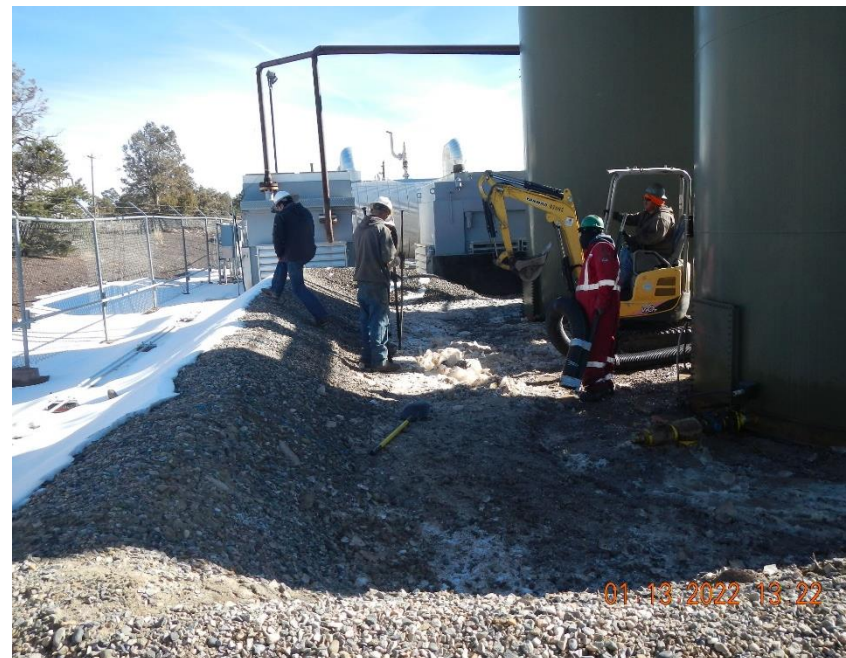
Personnel removing ice from within secondary containment berm.
