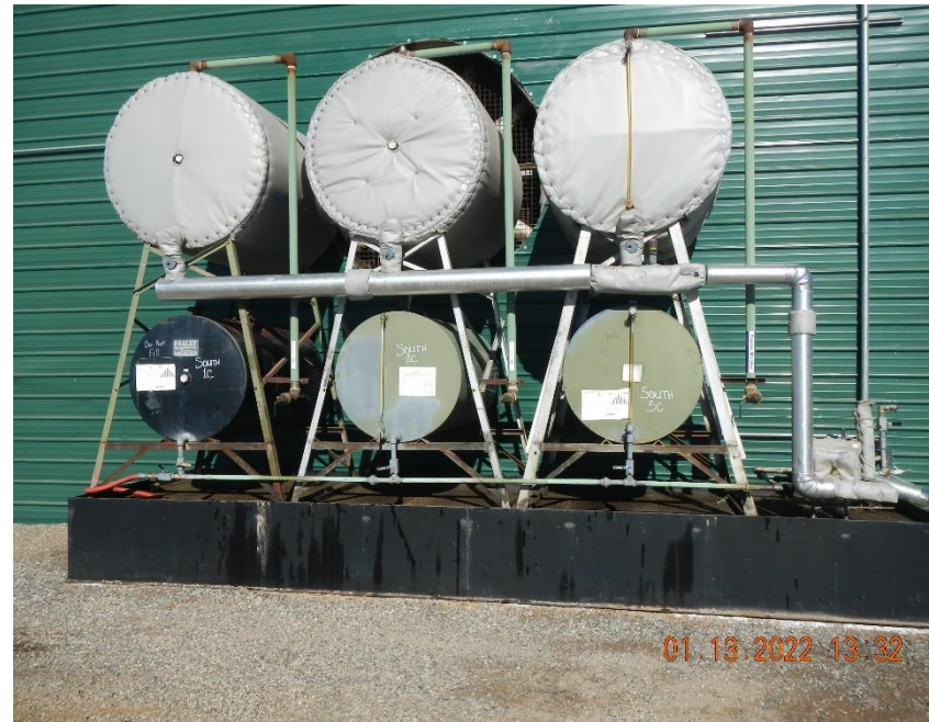
Secondary containment for lube oil containers.
