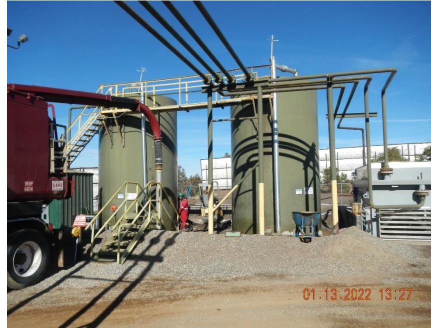
Personnel removing impacted material from within secondary containment berm.
