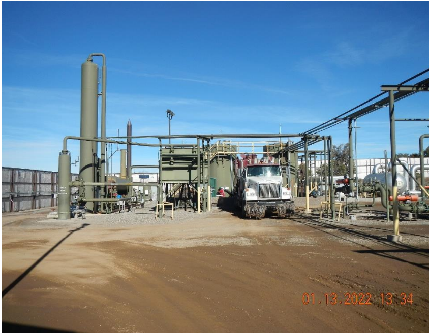
Hydrovac truck on site removing impacted material.
