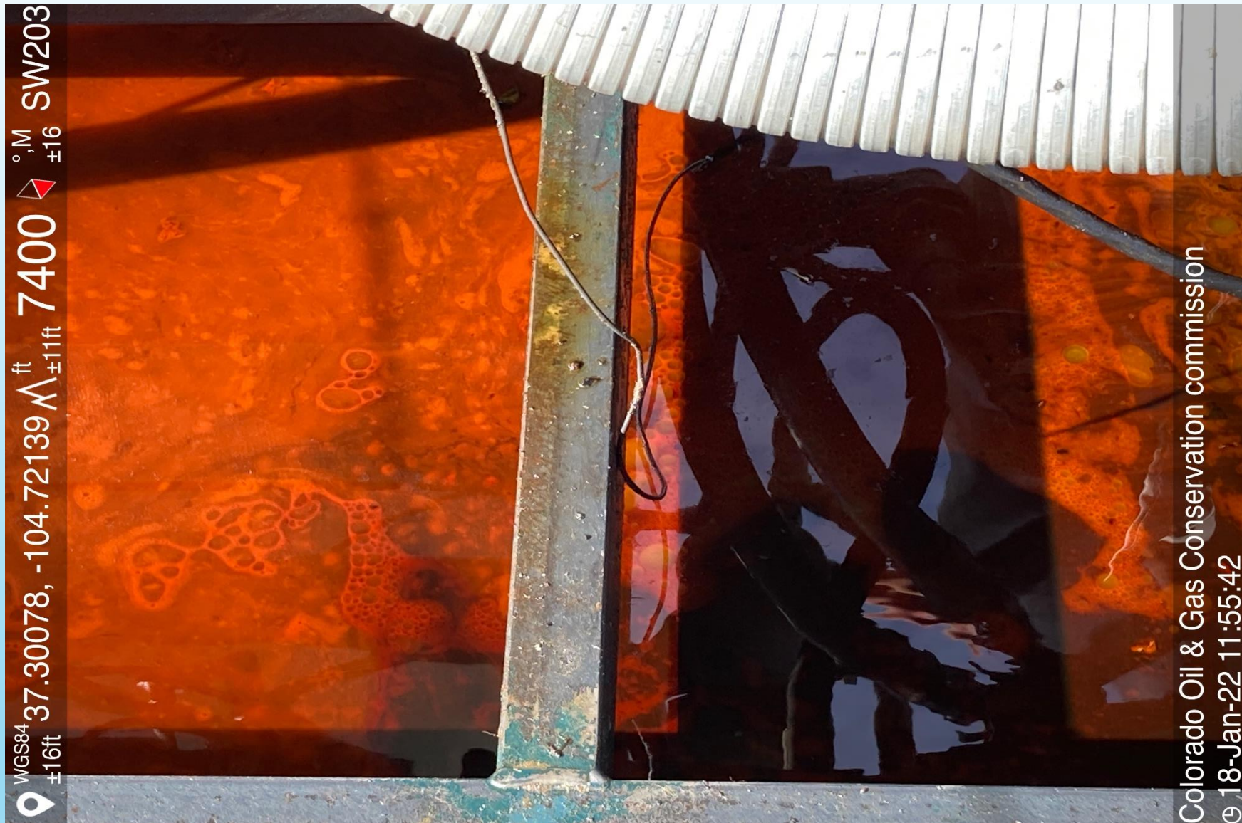
PHOTO 4: OILY WASTE IN COMPRESSOR POWER UNIT ENGINE SKID. COMPLY WITH RULE 1002.f.(2)B, Comply with general provisions of the oil and gas act for wildlife protection AND SB-181. CA DATE 1-19-2022.
