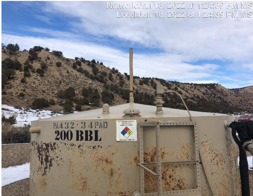
Photo #5717 Vent pipe on tank open ended.
