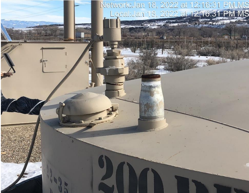
Photo #5707 Vent pipe on tank open ended.
