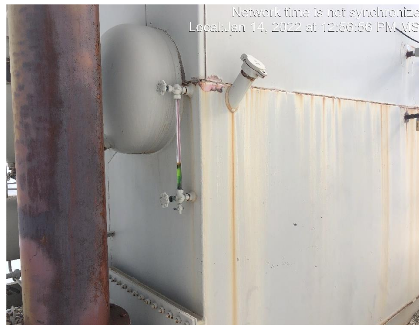
Photo #5700 Sight glass indicates the storage tank is full of an unknown fluid.
