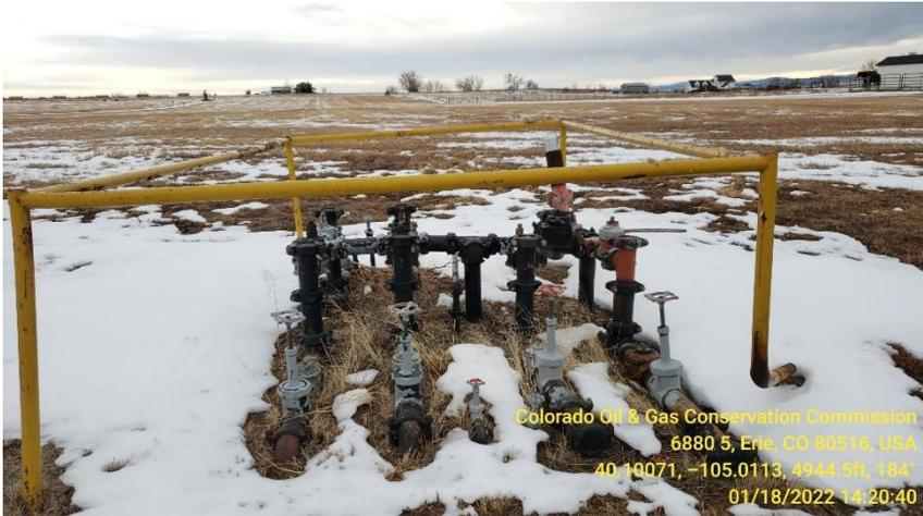
Photo 7 flow line manifold
