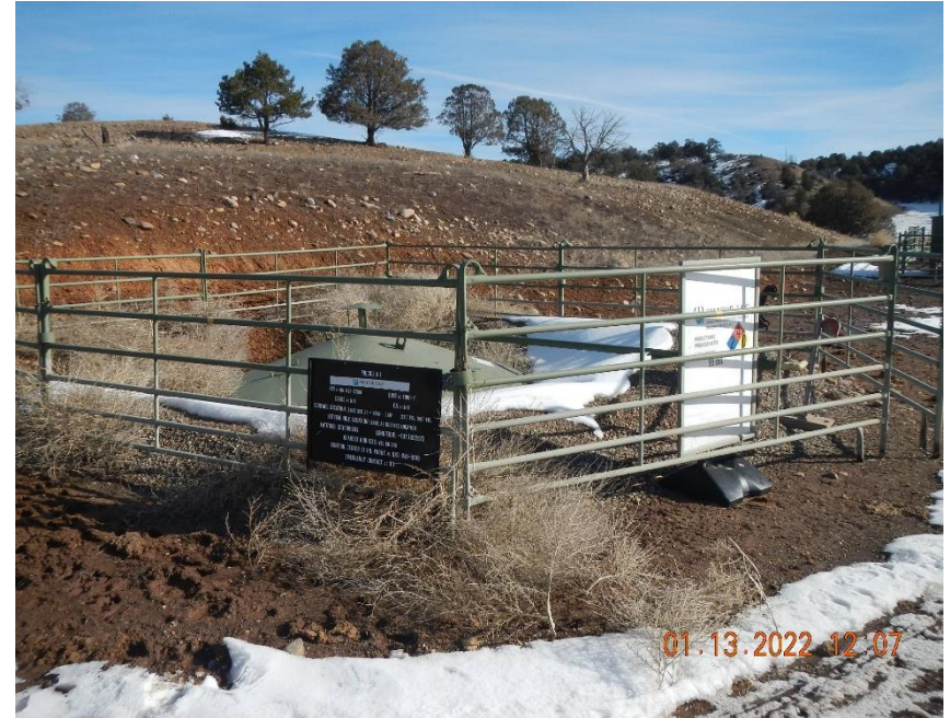
95 bbl. produced water PBV near location entrance.
