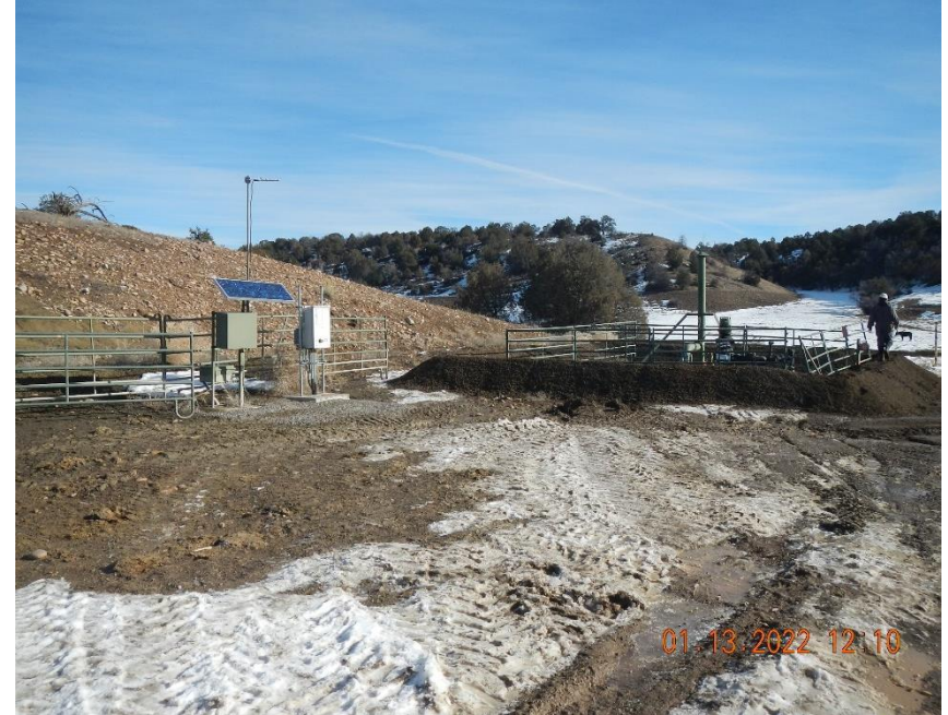
Earthen berm being constructed around double walled produced water PBV.
