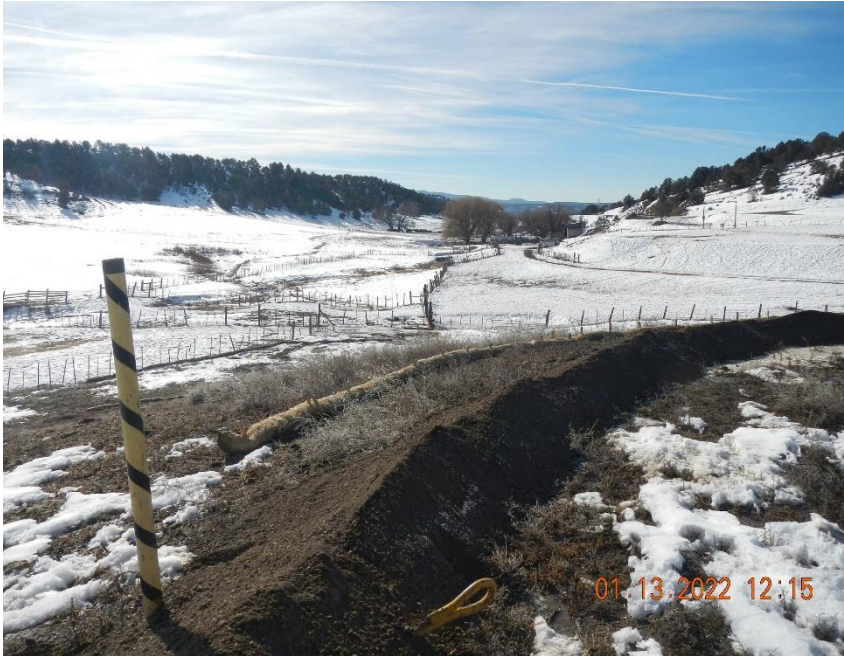
Recently installed perimeter berm. Wattles on SE corner of fill slope in response to Spill/Release Point ID #481402.
