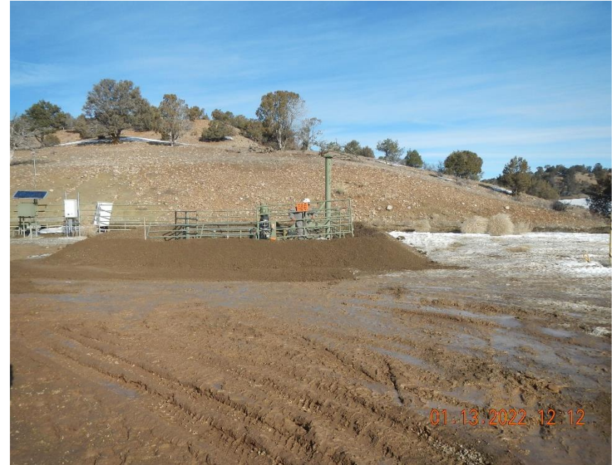
Earthen secondary containment berm around double walled steel PBV.
