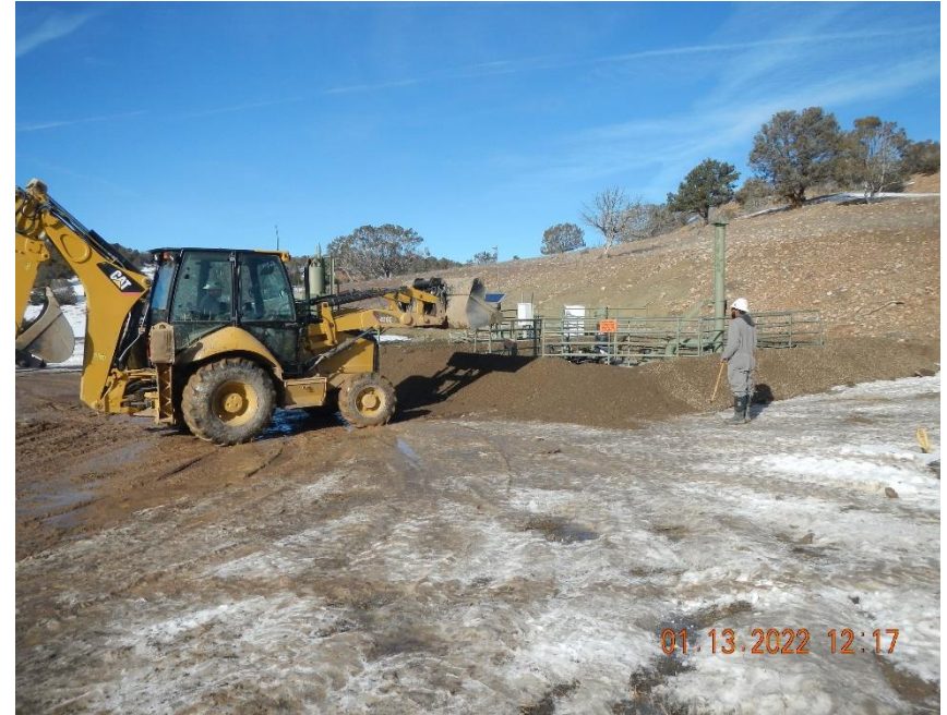
Earthen berm being constructed at the time of this inspection.
