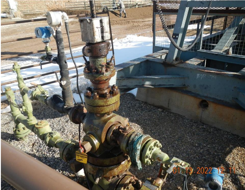
Well head is wet and stained.
