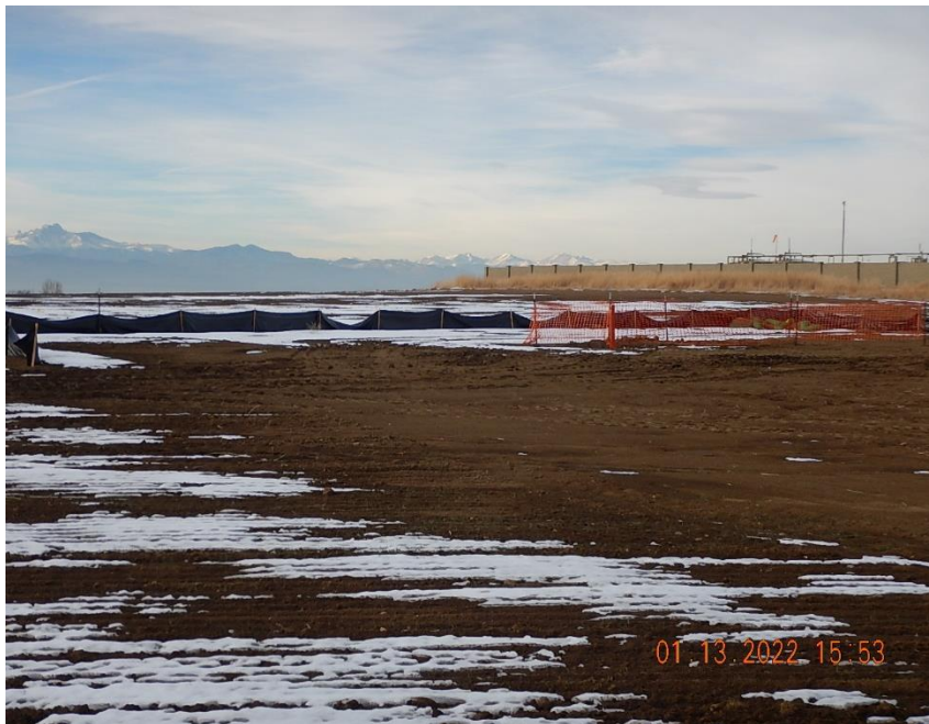
Firecracker consolidated flowline spill release area; view NW.
