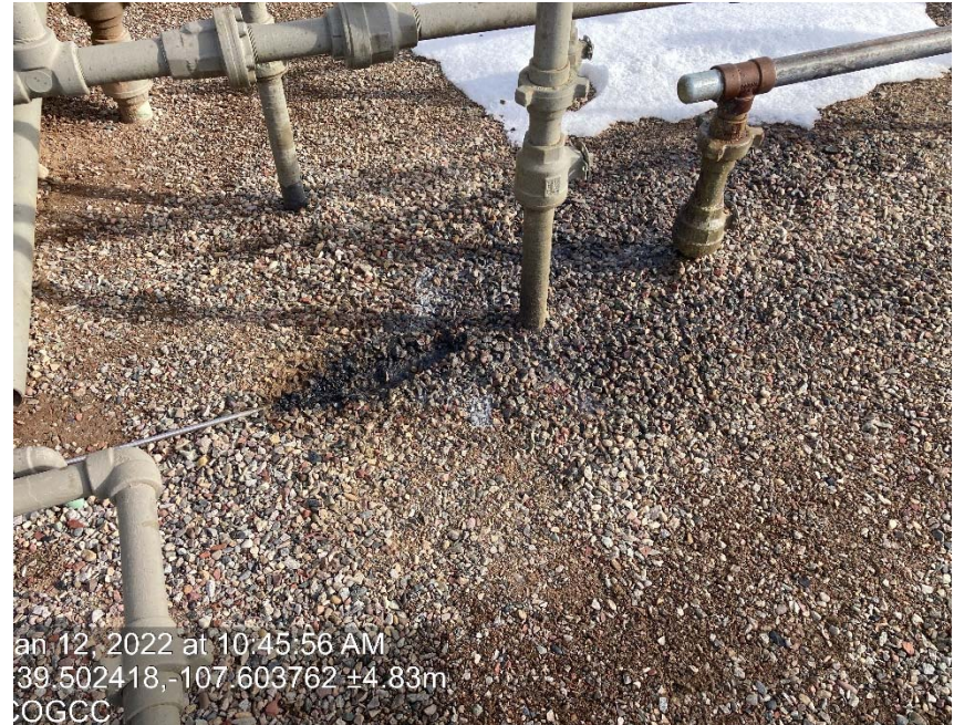
Staining from Trace pump exhaust
