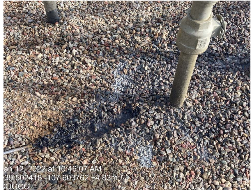
Staining from Trace pump exhaust
