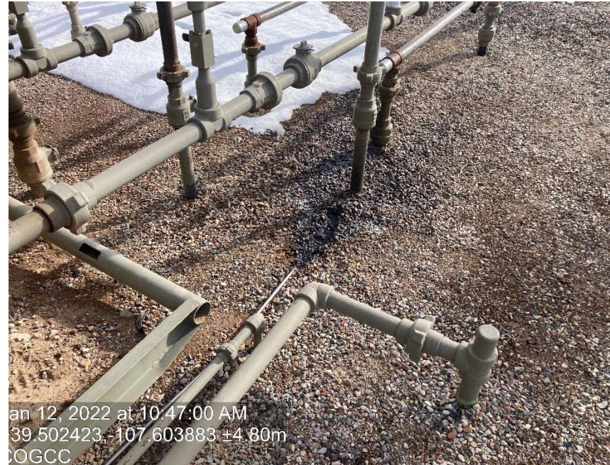
Staining from Trace pump exhaust
