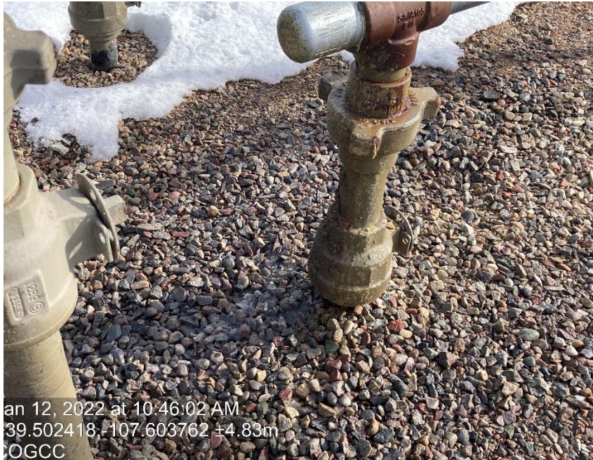
Staining from Trace pump exhaust
