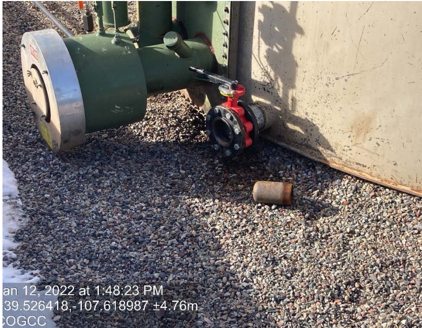
Load line missing cap/bull plug
