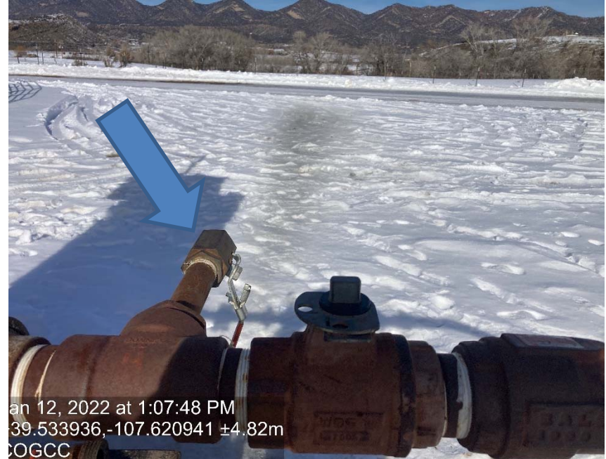
Staining/blow out valve from where the staining came from
