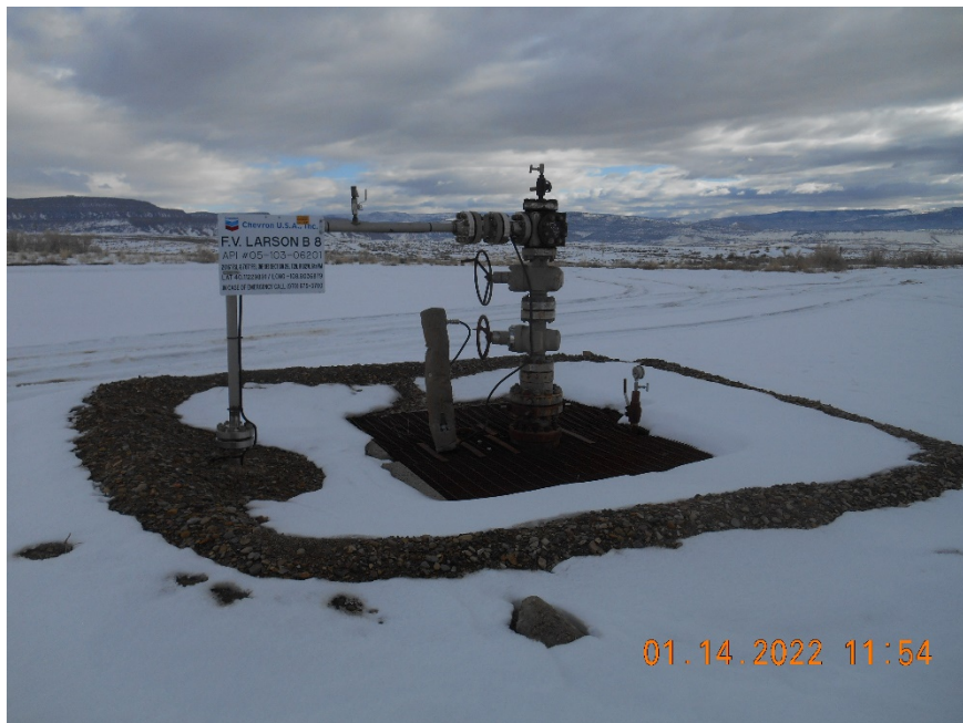
Injection wellhead
