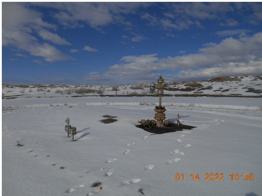
Injection wellhead – Temporarily abandoned
