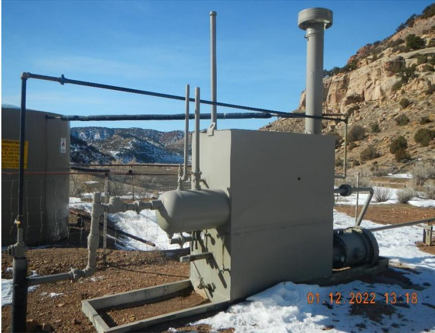
**No form of labeling or markers are present to identify a potential hazard or the contents of the storage tank.**
