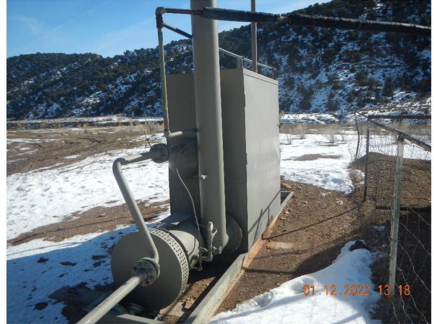
**No form of labeling or markers are present to identify a potential hazard or the contents of the storage tank.**
