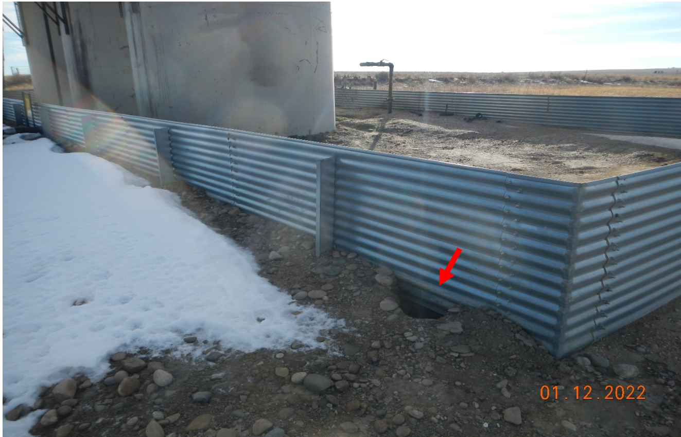
Photo 3. There is a hole at the outside edge compromising the secondary containment of the tank battery. Previous corrective action was not completed.
