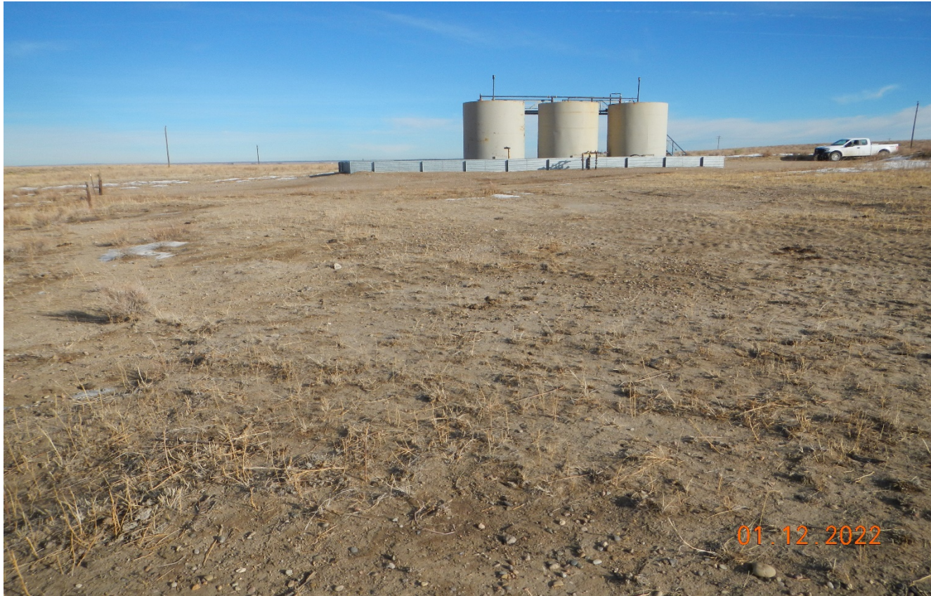
Photo 4. Facing north toward the tank battery. The area of disturbance south of the tank battery is bare of vegetation with compacted soils. This area needs to be reclaimed. Previous corrective action was not completed.
