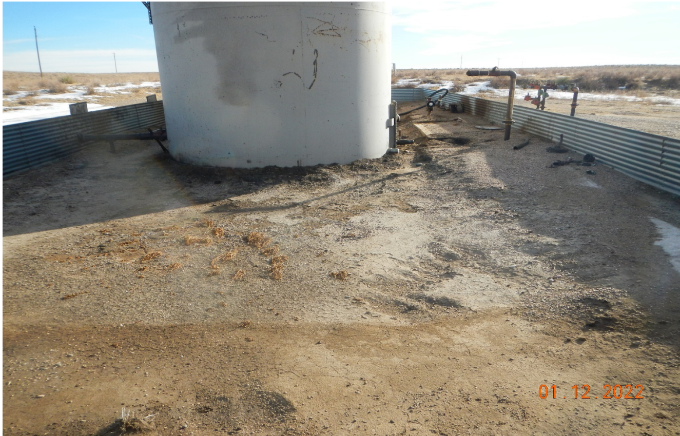
Photo 2. There is oil stained soil around the tanks which need to be cleaned up. Previous corrective action was not completed.
