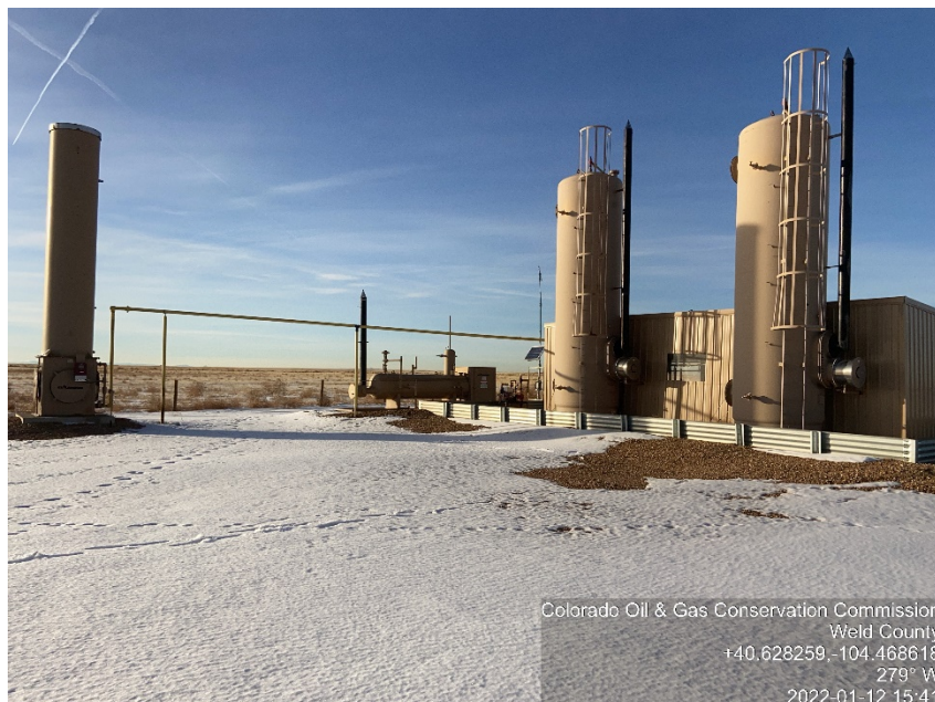
Photo #3 Bethyl GW 30-09 Tank Battery / Battery site Inactive / Shut-down ECD, Separator, Treaters
