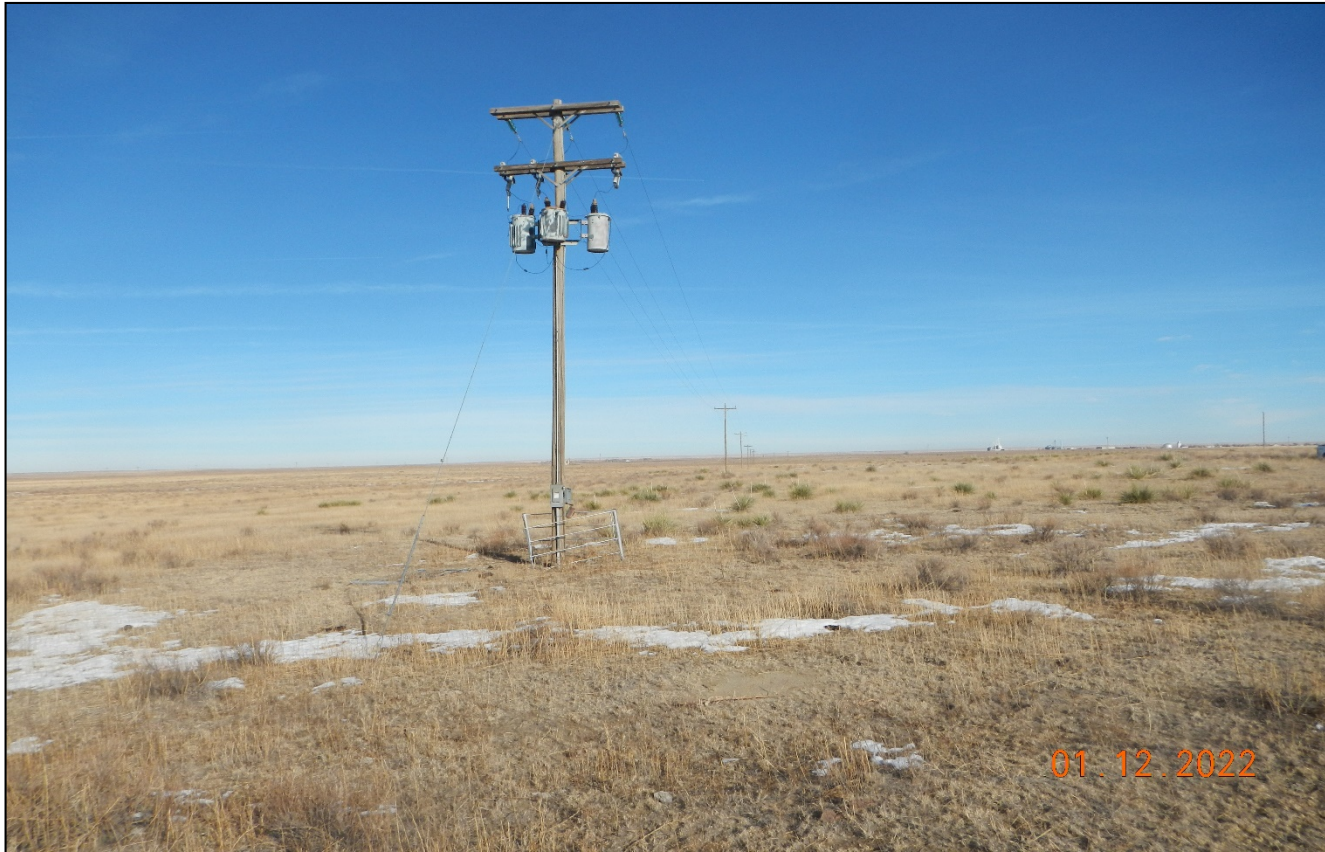
Photo 3. The powerline used for operating the well dead ends at the location and the entire unused portion of the powerline must be removed.
