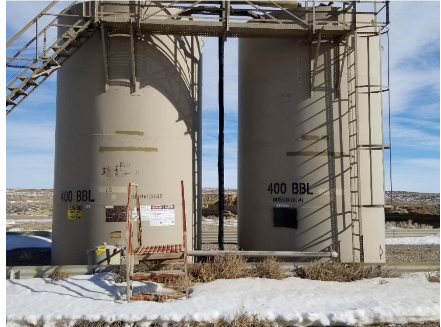
Photo 2. Tank labels faded/missing.
