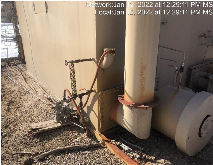
Photo #5667 Sight glass indicates the storage tank is full of an unknown fluid.
